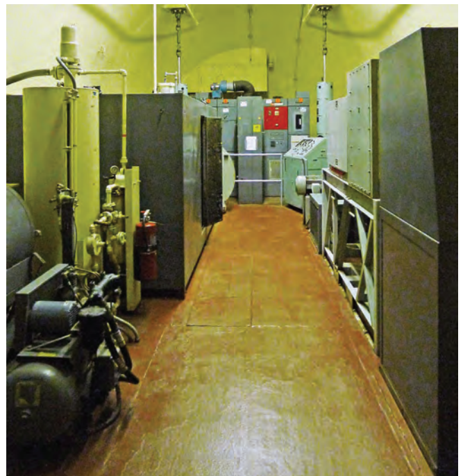
LCEB Interior view
